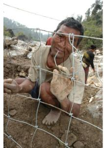
Figure 5: Making gabion cages by hand with a square mesh.
