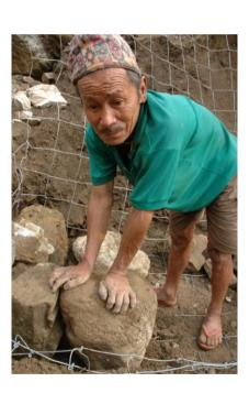
Figure 12: Loading rocks into the gabion cages, a community activity. Photo: Practical Action Nepal.
