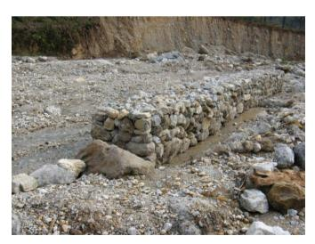
Figure 6: An example of a spur that has not been installed with groundwork or an apron and consequently is likely to be washed away during heavy flooding.
