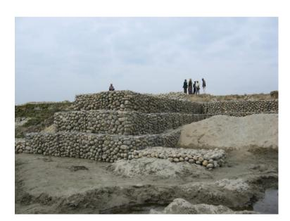
Figure 4: A newly constructed spur shown before the monsoon. The base of the river and the spur apron are clearly visible in the dry season. Photo: Practical Action Nepal.
